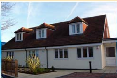
"Good" - CSCI Inspection Report - April 2008
